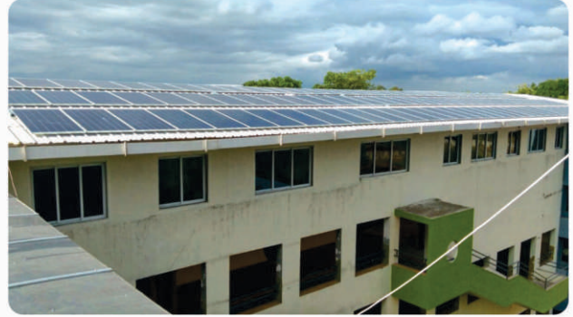
32.5KW Solar Power Plant Anand Niketan - Shilaj
